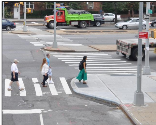
Curb Extension/Bump-out/Neckdown
