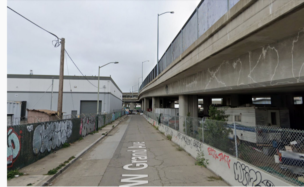
West Grand Alley Elevation Today (view West)
