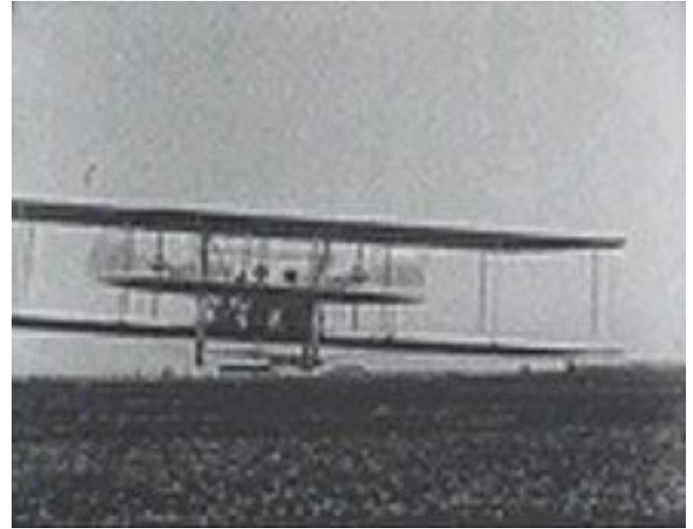
Building the first airplane
